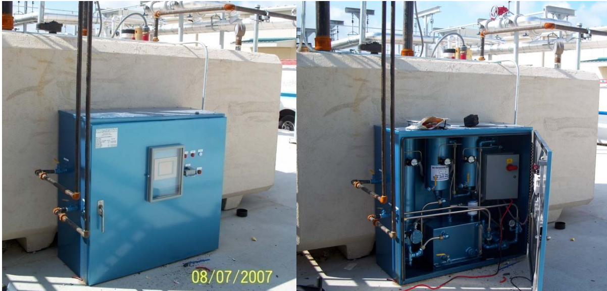
Enclosed Diesel Generator Fill and Polishing System from Main Tank to Generator Belly Tank Specifications: 8 GPM, Touch Screen, Pre and Post Filtration with Fuel Water Separator / Coalescer.
